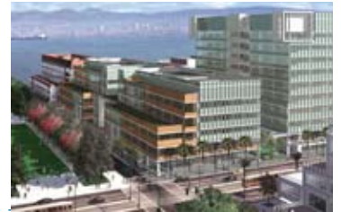
455 Mission Bay Boulevard is located in the current hotbed of the biotechnology industry.
