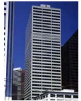
One of the largest sublease blocks recently created is located at 45 Fremont Street
